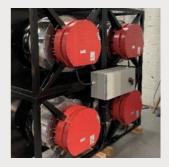
Aircore EC motor mounting secures all four sides of the motor. Front-to-back spacing must accommodate the size (i.e., depth) of the wheel.
